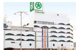
Shimonoseki Daimaru (Floor space: 23,912m 2 )
