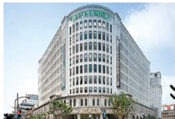
Daimaru Kobe (Floor space: 50,656m 2 )
