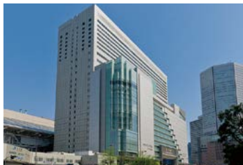
Daimaru Osaka Umeda (Floor space: 64,000m 2 )
