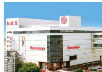
Matsuzakaya Toyota (Floor space: 18,220m 2 )
