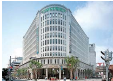
Daimaru Kobe (Floor space: 50,656m 2 )
