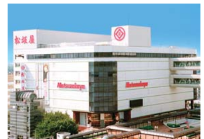
Matsuzakaya Toyota (Floor space: 18,220m 2 )
