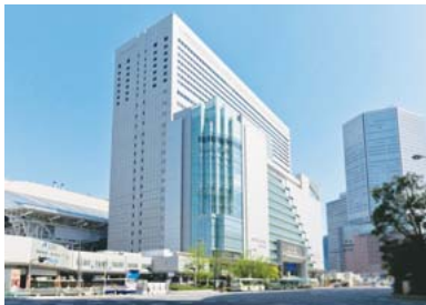
Daimaru Osaka Umeda (Floor space: 64,000m 2 )
