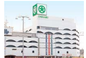
Shimonoseki Daimaru (Floor space: 23,912m 2 )
