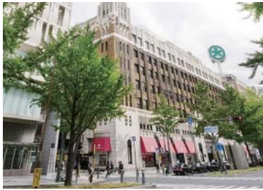
Daimaru Osaka Shinsaibashi (Floor space: 77,490m 2 )
