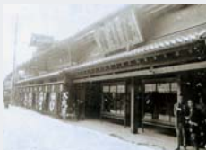
Show windows of Osaka store that first appeared in Osaka in 1914
