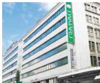
Daimaru Kyoto (Floor space: 50,830m 2 )
