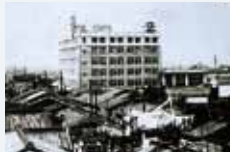
Osaka store whose first phase of construction was completed in 1922
