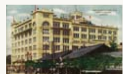
Nagoya store moved to the present location in Minamiotsumachi (at that time)
